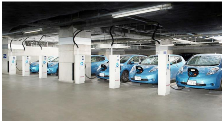
Figure 3:5: Fleet of Nissan Leafs being used as V2B resources to power an office in Japan 5
