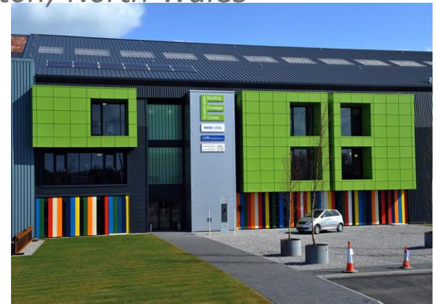
TATA Sustainable Building Envelope Shotton, North Wales
