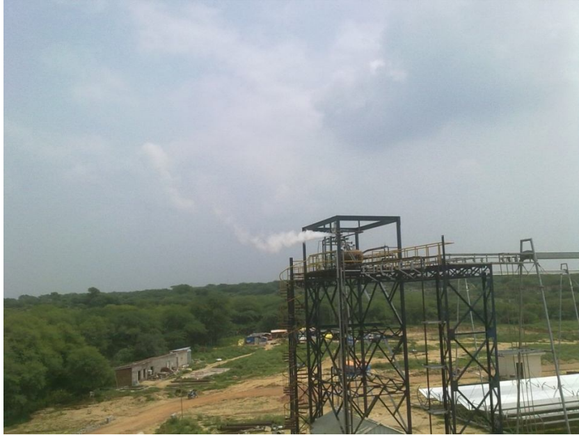
Fig 27: The steam generated by the LFR solar Field, during testing.
