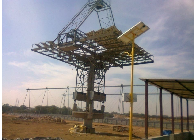
Fig 14: Arun Dish installed
