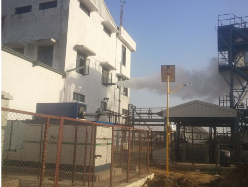
Fig 30: Steam blow off at 44 Kg/cm 2
