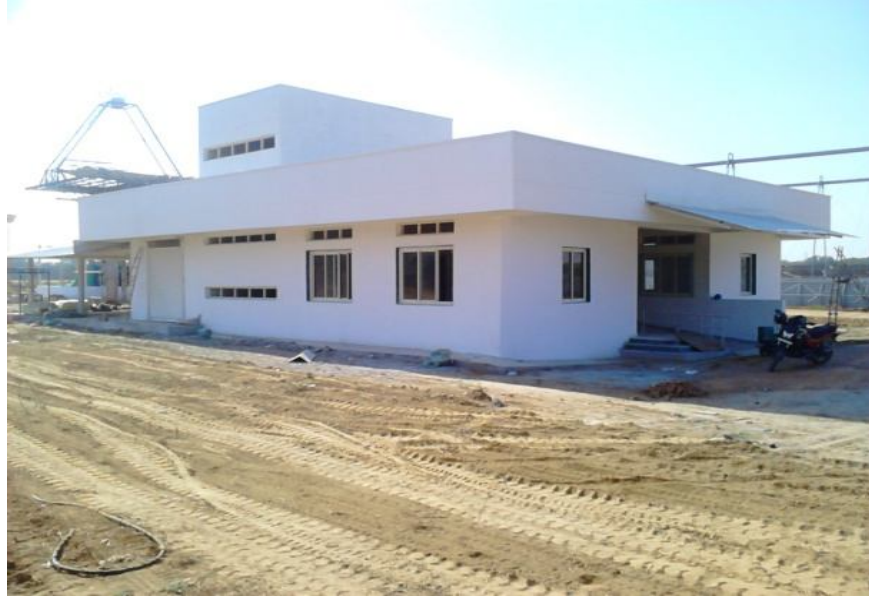
Fig 12: Testing Rig Building
