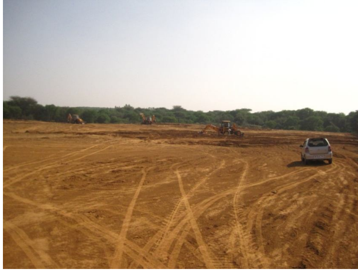
Fig 23: Leveling of Site.
