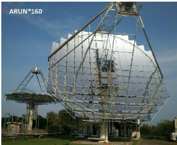
Two dishes of ARUN160 for 50TR space cooling with pressurized water system at 10 bar(g) at Turbo Energy near Chennai
