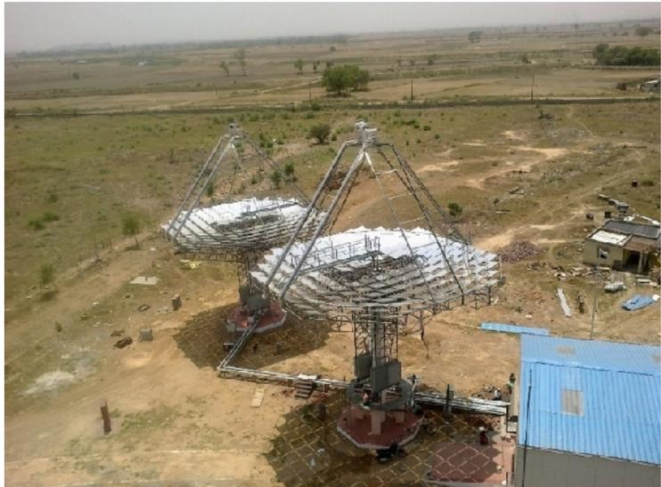
Two dishes of ARUN160 for 50TR space cooling with steam system at 10 bar(g) at NETRA, NTPC, Greater NOIDA near Delhi
