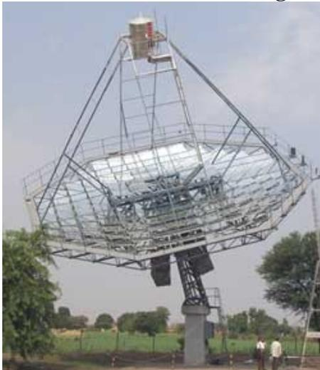
ARUN 160 at Mahananda Dairy supplying heat anytime of the day with pressurized water storage at 20 bar(g) installed and commissioned in 2006 and smoothly operating till now
