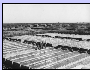
5000 lpd solar distillation plant
